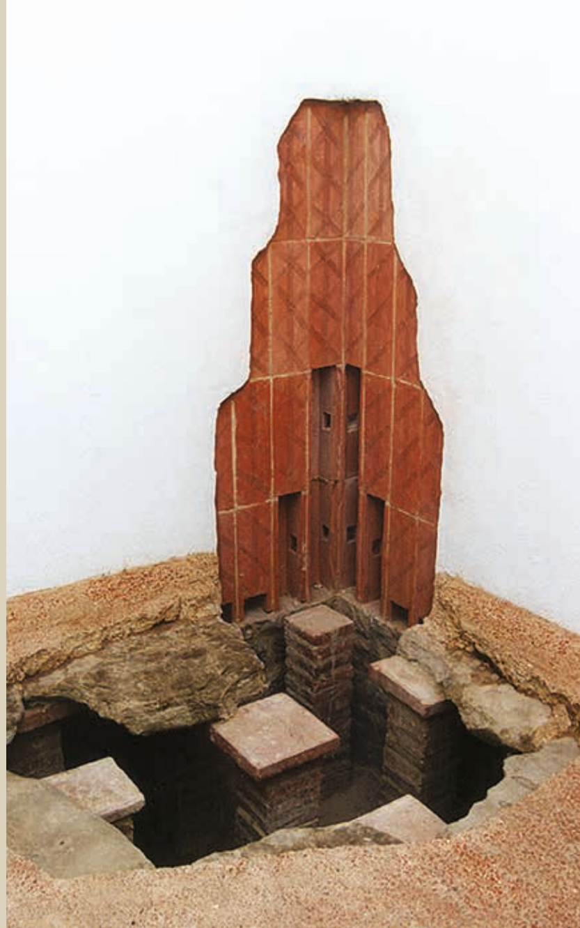
How the baths worked - underfloor heating and flues in the walls (in the reconstructed baths at Segedunum)
