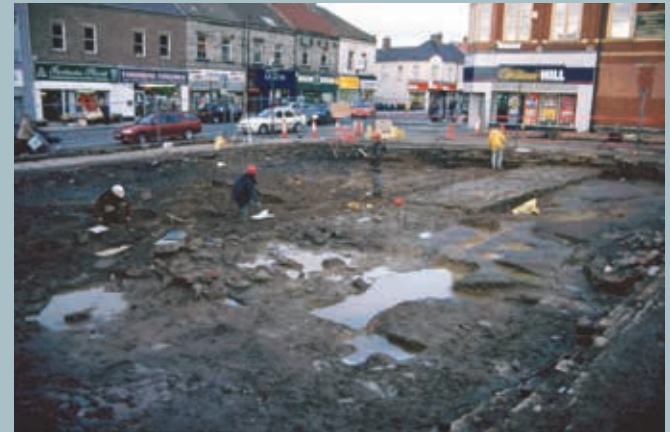
The foundations of the Narrow Wall revealed on the south side of Shields Road, Byker, in 2000
