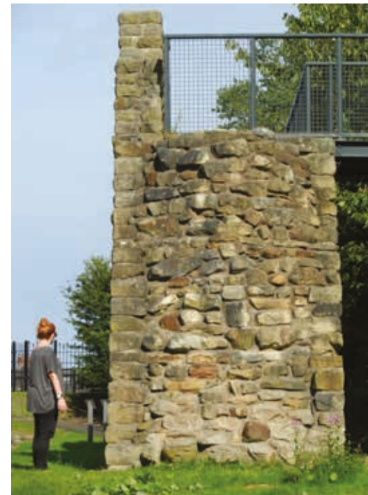
Right: Reconstruction at Wallsend-Segedunum showing cross section through the Wall as it would have appeared originally
